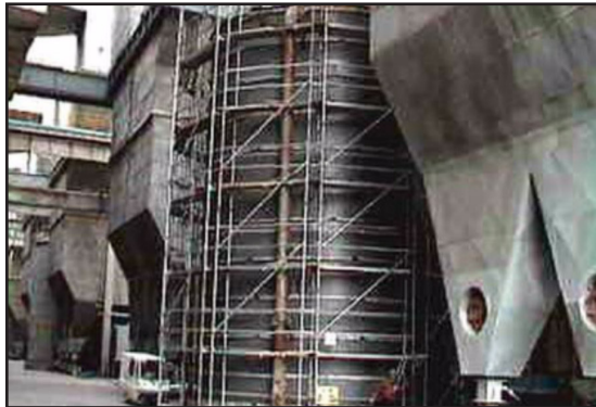
Outside view of one of the tanks
